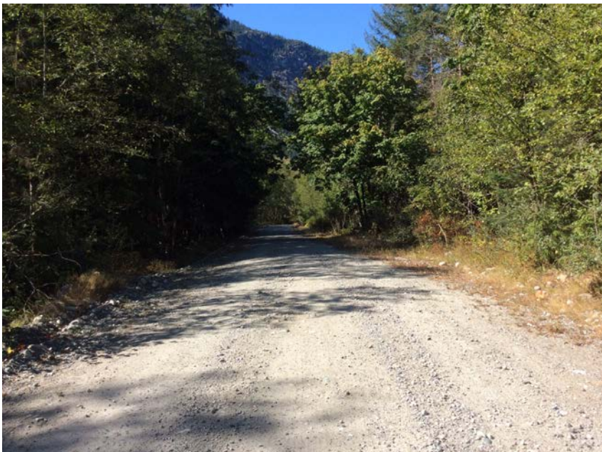
Right approach viewed from bridge
